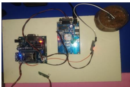
Fig. 9. Base Station (Landslide site)
