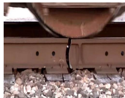
Fig. 1. Rail crack track
